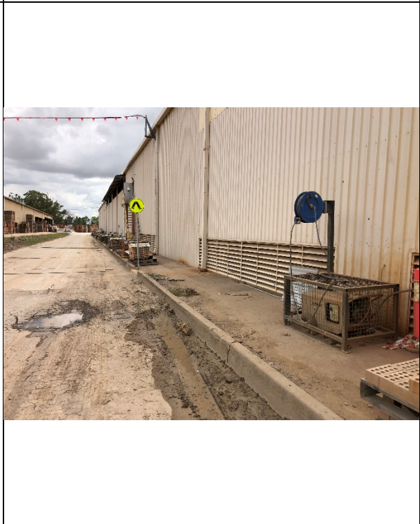
Picture 56: IMG_5950 Wheel wash hose
