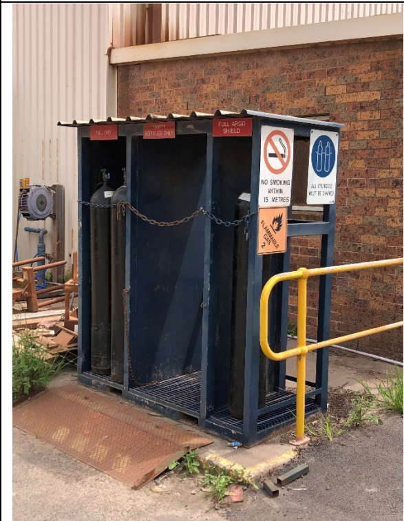
Picture 59: IMG_5954 Gas storage
