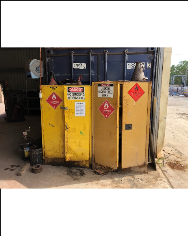
Picture 30: IMG_5907 Flammable liquid storage
