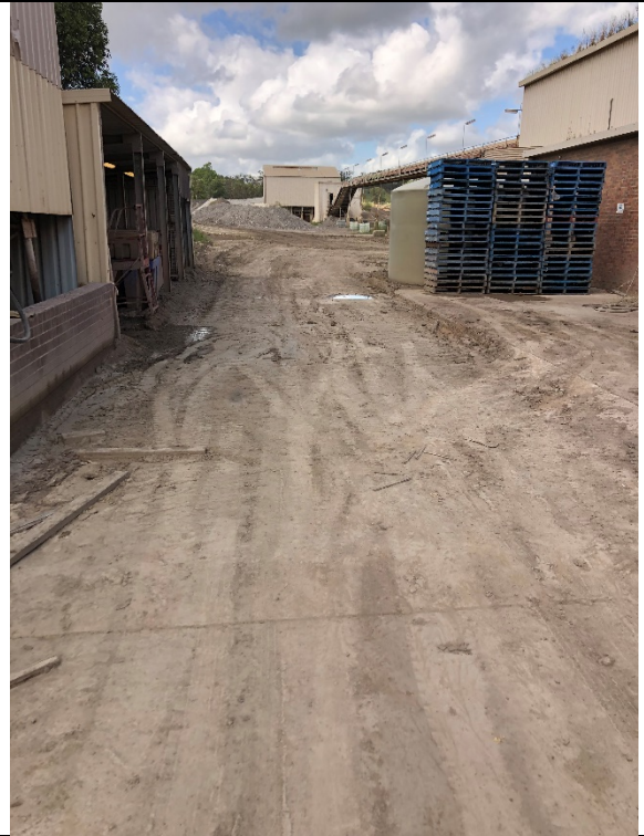
Picture 26: IMG_5903 Bunded driveway at fuel stations
