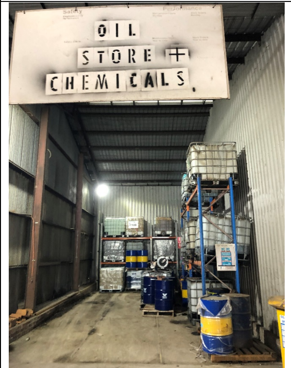
Picture 63: IMG_5959 Bunded oil and chemical storage
